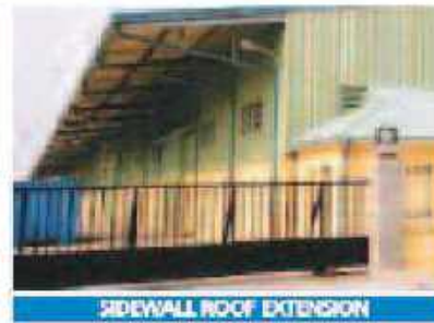
SIDEWALL ROOF EXTENSION
